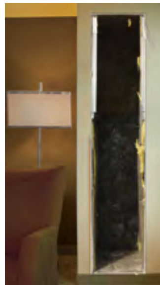
Remove internal components and trim cabinet edges.
