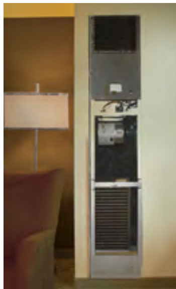
Remove surface components and trim drywall.
